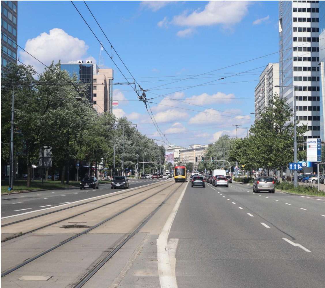
Jana Pawła II Avenue in July 2020 north of ONZ roundabout where the roadway is six lanes-wide, with short side-lanes for diagonal parking. The tramway line runs in the median without any separator. Sidewalks are narrow and show little urban activity. © Cybularny
