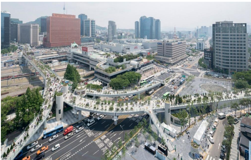
The Sky Garden in Seoul (Korea): a former fragilized road viaduct recycled as a green pedestrian Connection to the Central Station MVRDV © Ossip van Duivenbode
