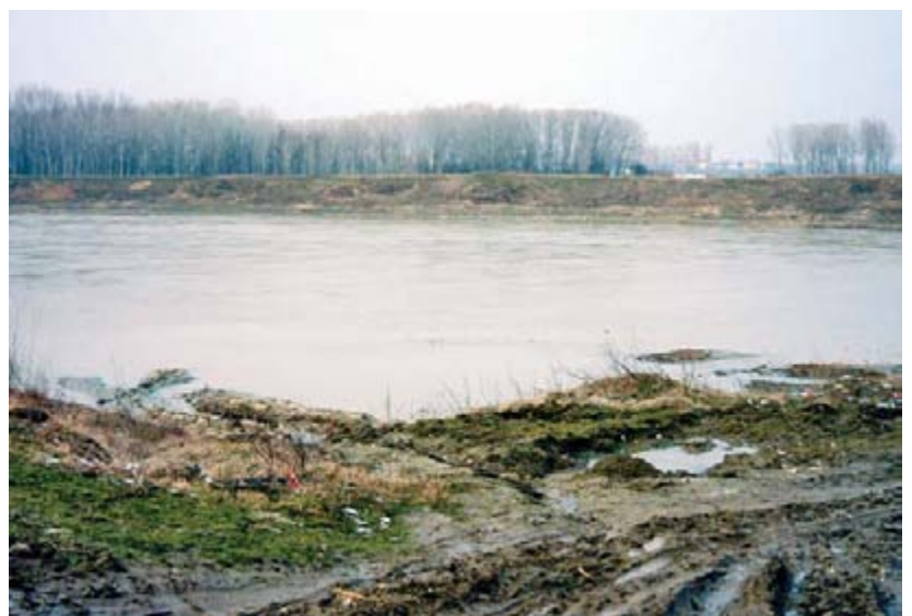
Picture 29 The Existing Stage of works at The Bucharest – The Danube River Navigable Channel.
