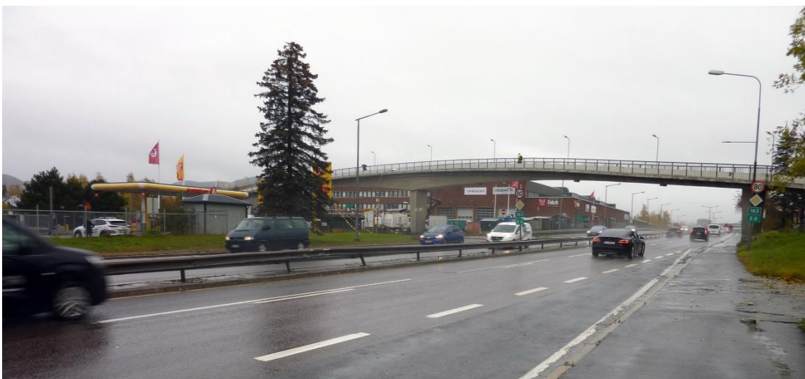
Østre Aker vei road environment seen from a pedestrian point of view
