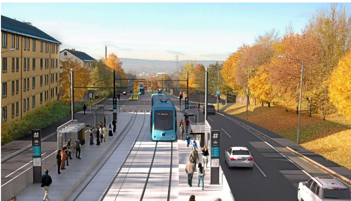
Trondheimsveien boulevard transformation project, with construction of a tram line in a widen median (2014)
