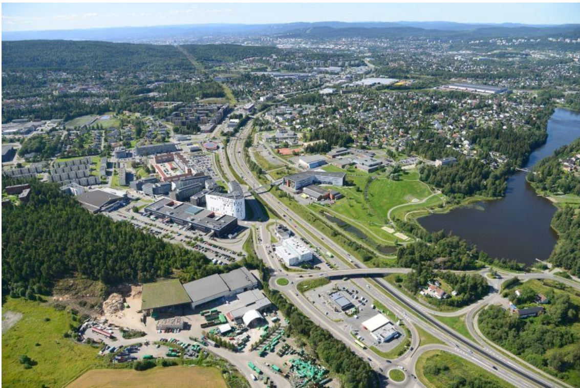
Residential and commercial car-oriented land use in Akerhus. Lørenskog along the highway to Lillestrøm
