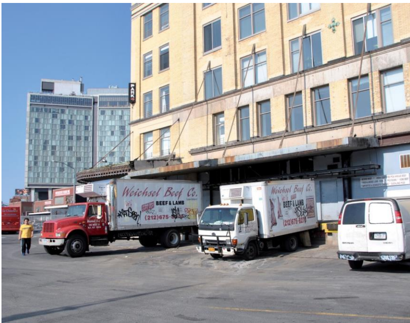
Refrigerated warehouses in the Meatpacking District in 2011 along the West Side Avenue © P. Lecoart IAU idF
