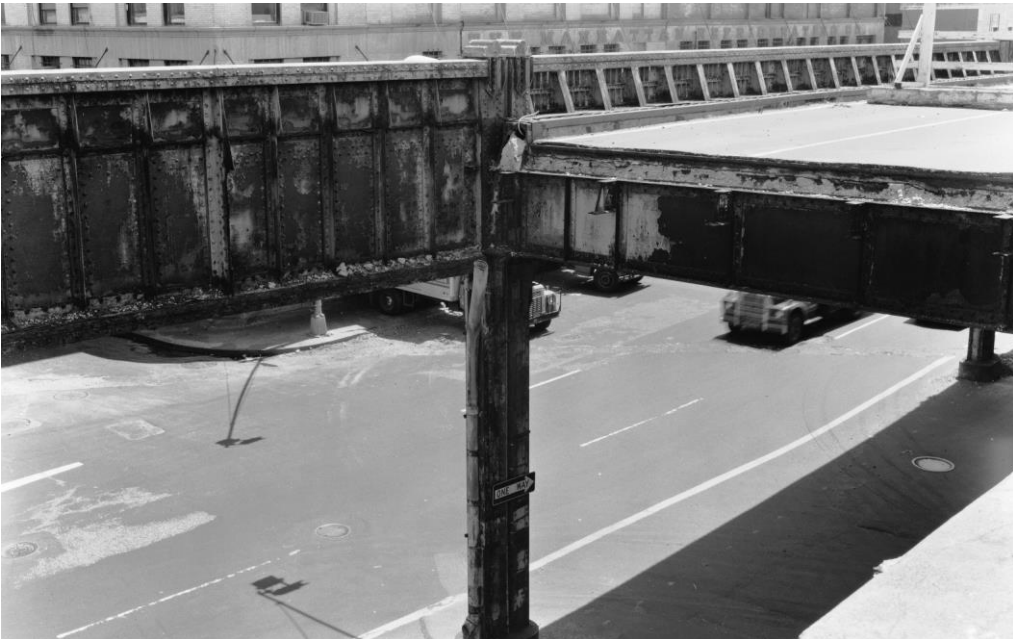
The collapse of the West Side Highway viaduct in 1973 due to lack of maintenance © Steven Zane/Library of Congress
