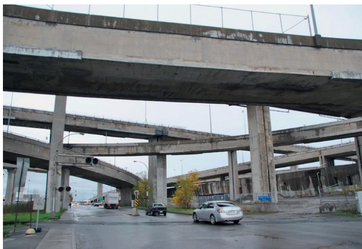
The Turcot Interchange, which connects the A-15, A-20 and A-720 highways, is currently under reconstruction. The CAN$3.7 billion project is expected to be completed by 2020. © P. Lacroart IAU idF
