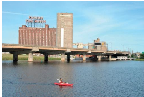
The Bonaventure Expressway as it crosses the Peel Basin.
