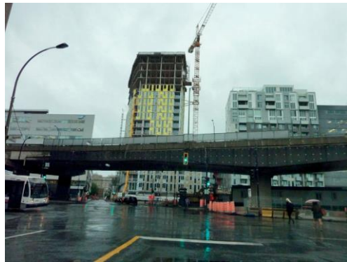
The highway's surroundings are becoming denser in anticipation of the project. New condominiums under construction in 2014. © P. Lecroart IAU îdF
