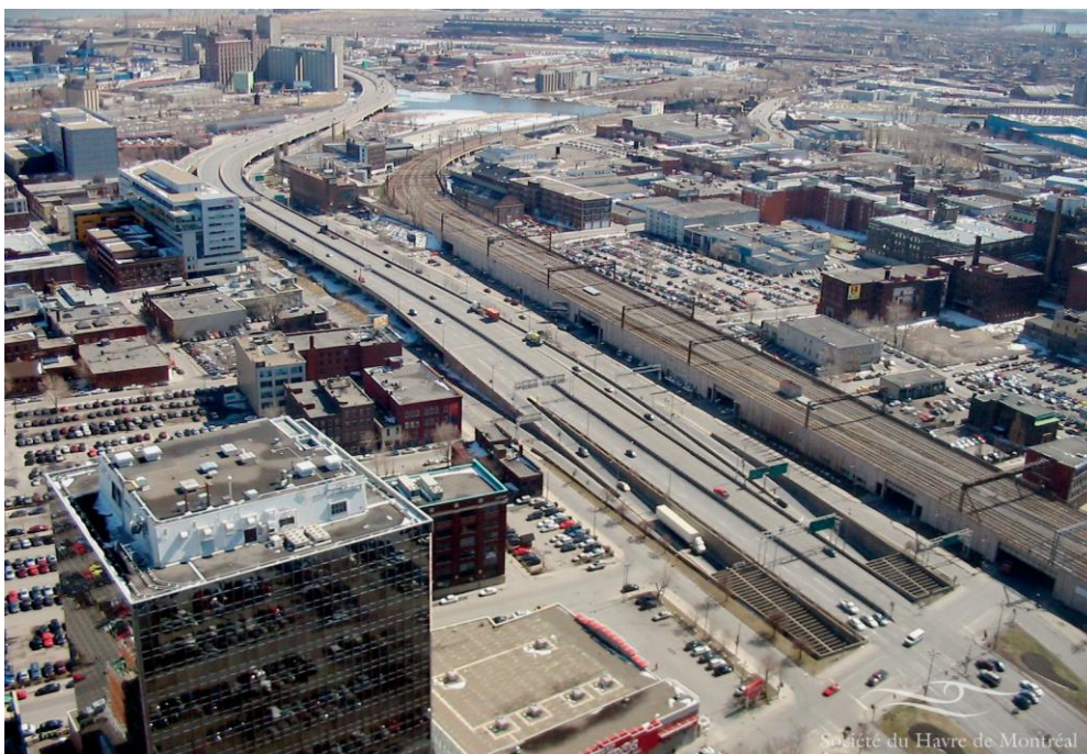
The Bonaventure Expressway and the Montréal Harbourfront seen from the business center: an urban divide between the Faubourg des Récollections (left) and the Griffintown district (right) © Société du Havre de Montréal
