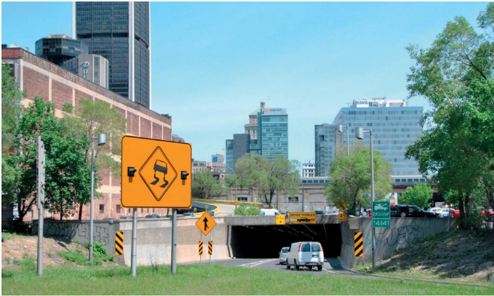
Access to the tunnel to the Ville-Marie Expressway from the Bonaventure district © P. Lecroart IAU idF
