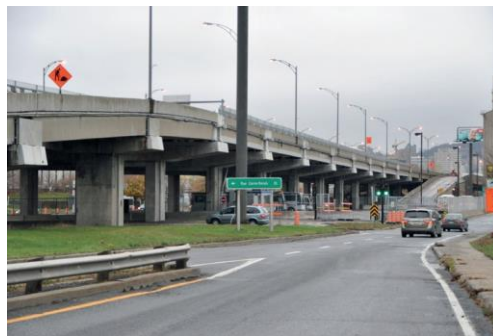
South of the Peel Basin, the highway is again a viaduct. The initial project was to transform this section during phase 3. © P. Lecroart IAU îdF
