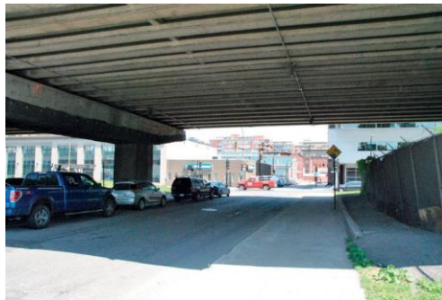
The highway and its viaduct create a strong urban divide south of the Montréal city center.
