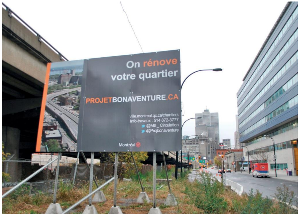
Construction begins: the Bonaventure Project in November 2012 © P. Lecroart IAU îdF
