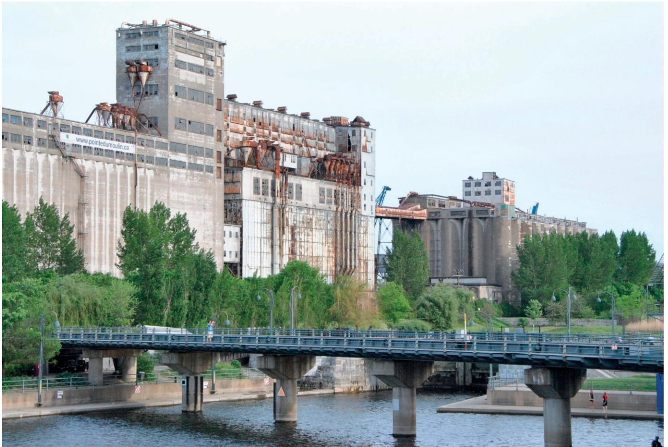
Grain Elevator No. 5 which will be converted, south of the Lachine Canal. © P. Lecroart IAU idF
