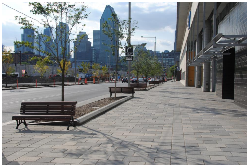
The new boulevard during the last construction phase (Summer 2017). © P. Lacroix IAU idF
