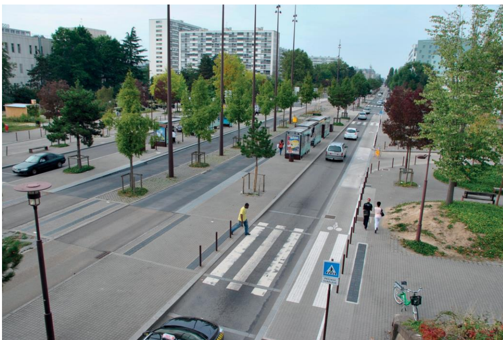
The urban avenue to replace the A801 highway in Nantes (Busway dedicated lane in the center). © P. Lecroart IAU îdF
