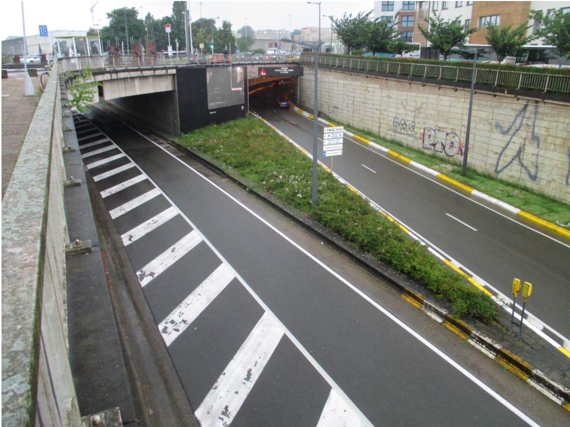
The E411 expressway trench at the Beaulieu metro station (left) is a major barrier between the municipalities of Auderghem and Watermael-Boitsfort. The Master Plan aims at filling in the trench to the right and reconnecting public space at ground level.
