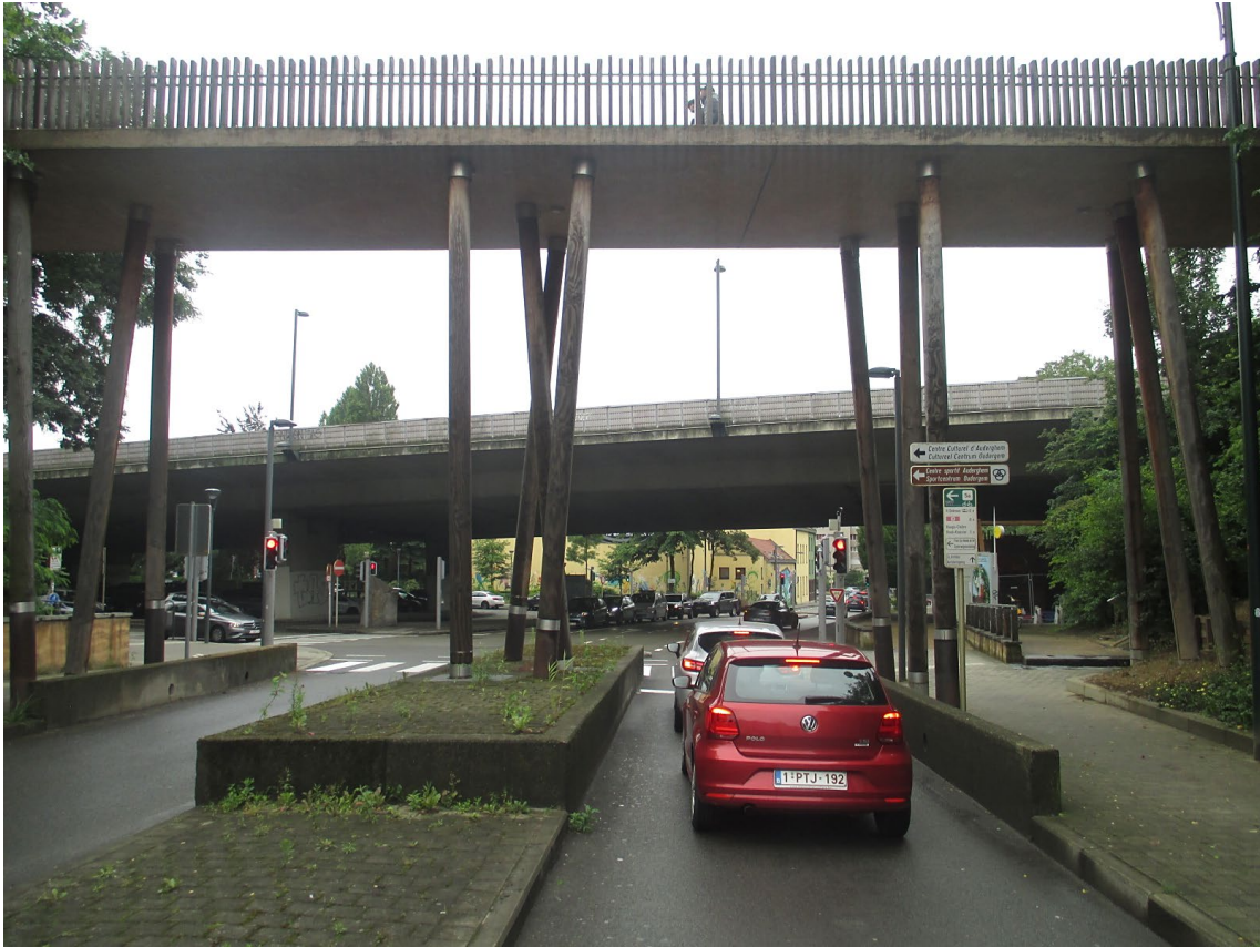
The Watermael Viaduct (in the background): a visual and partly physical barrier between neighbourhoods. © Paul Lecroart - L'Institut Paris Region
