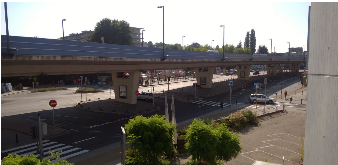
The Herrmann-Debroux Viaduct © Perspective.Brussels
