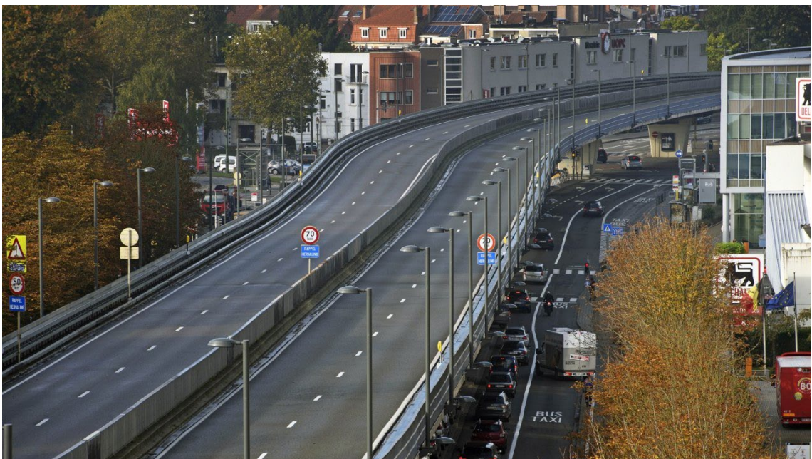
The Herrmann-Debroux viaduct after its temporary closure for inspection in 2017. © Le Soir
