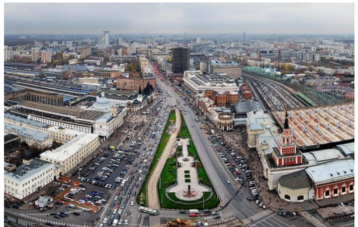
Three railway stations on Komsomolskaya Square - one of the centers of Moscow regional and federal passenger connections
